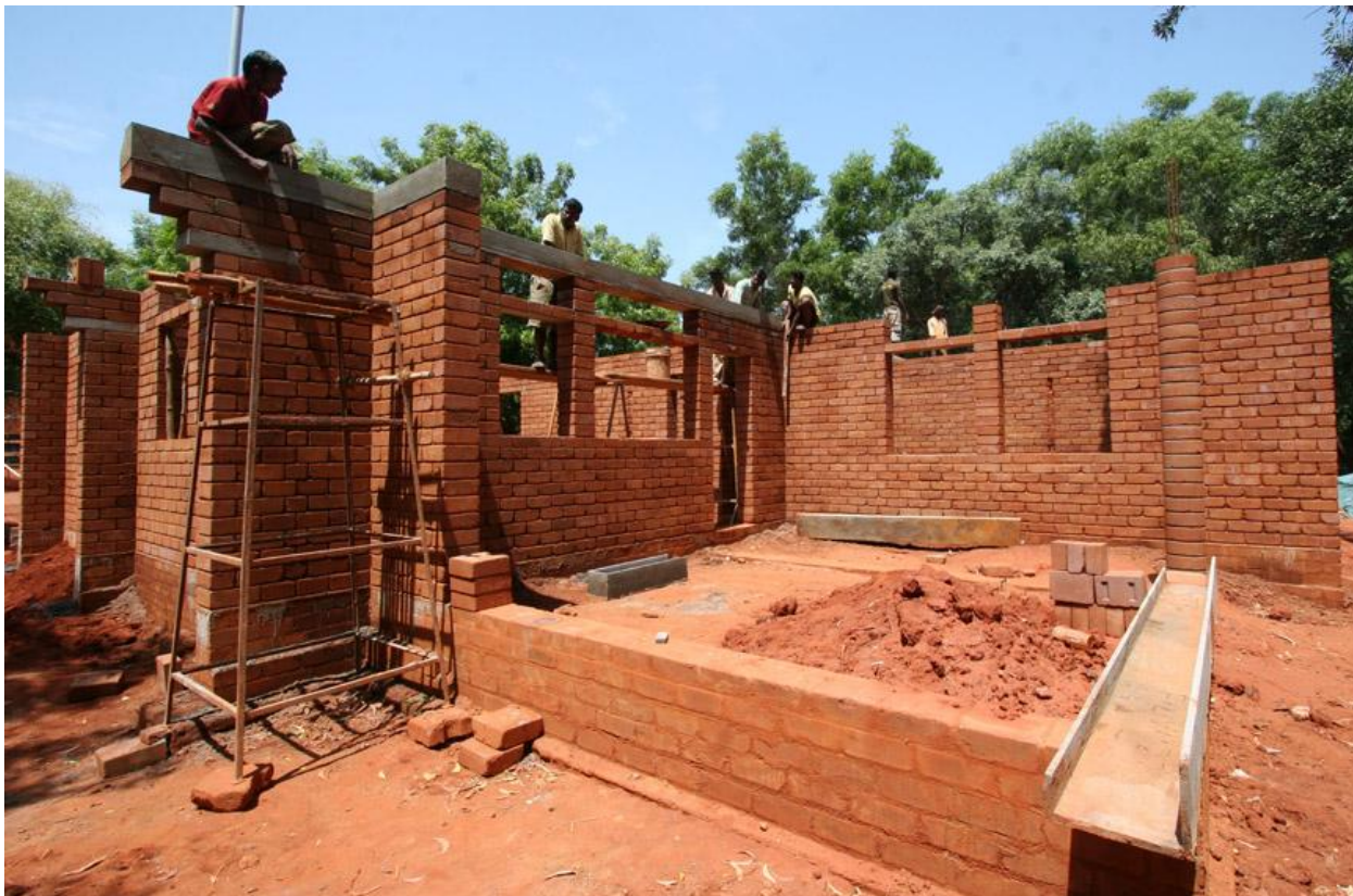
North Block under construction
