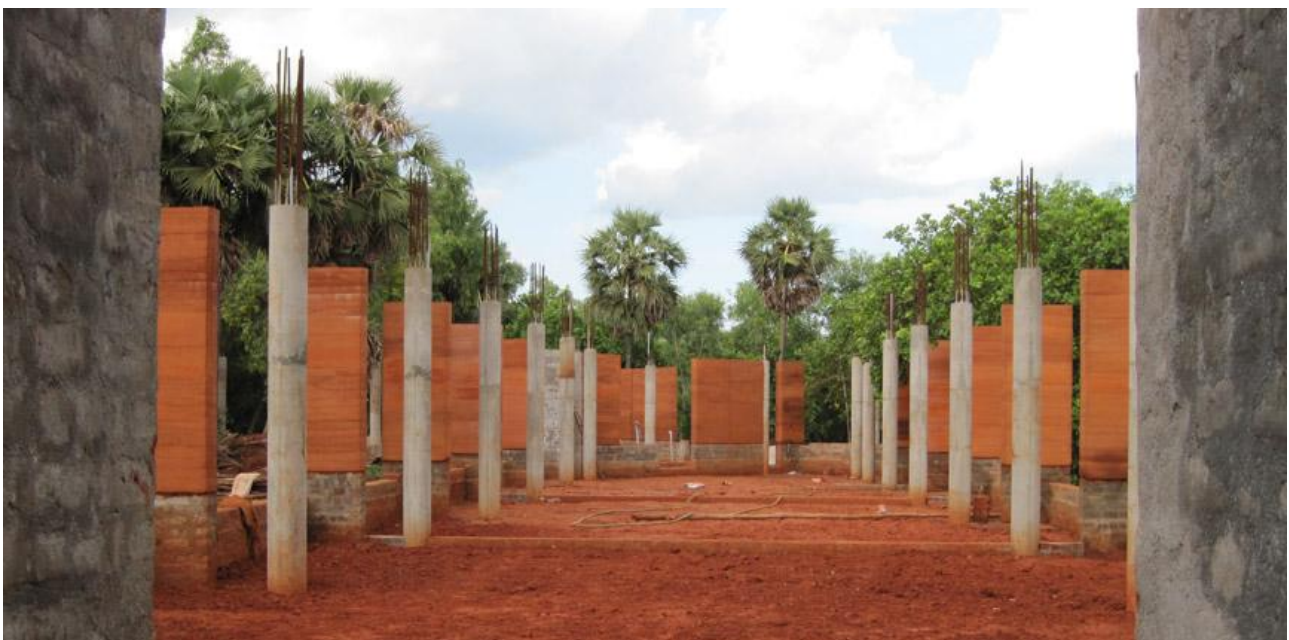
Works in progress ...
