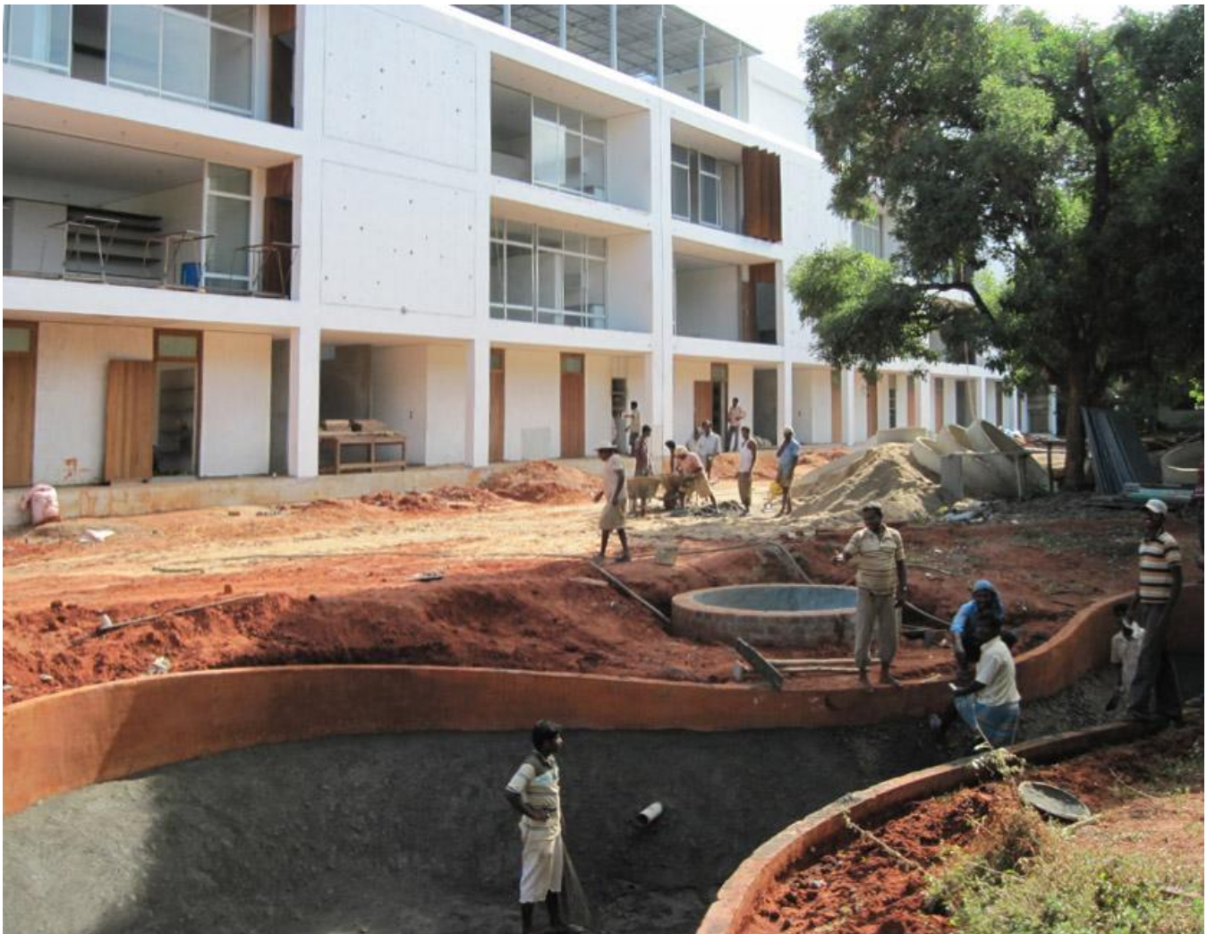
Works in progress ...
