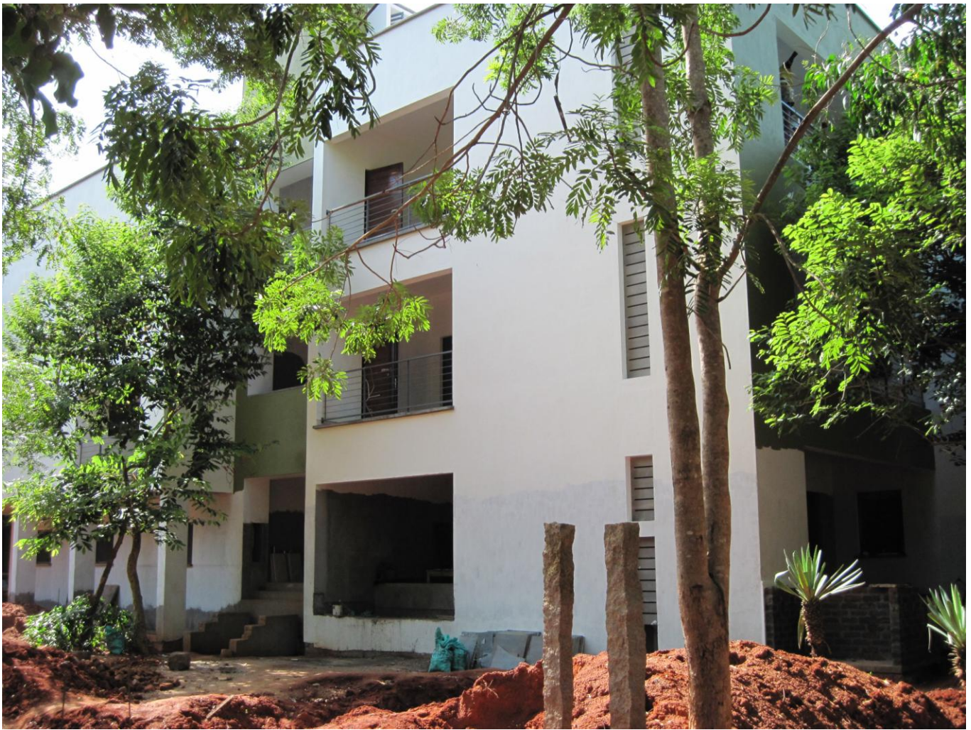
Arati III, Building 1: 95% completed
