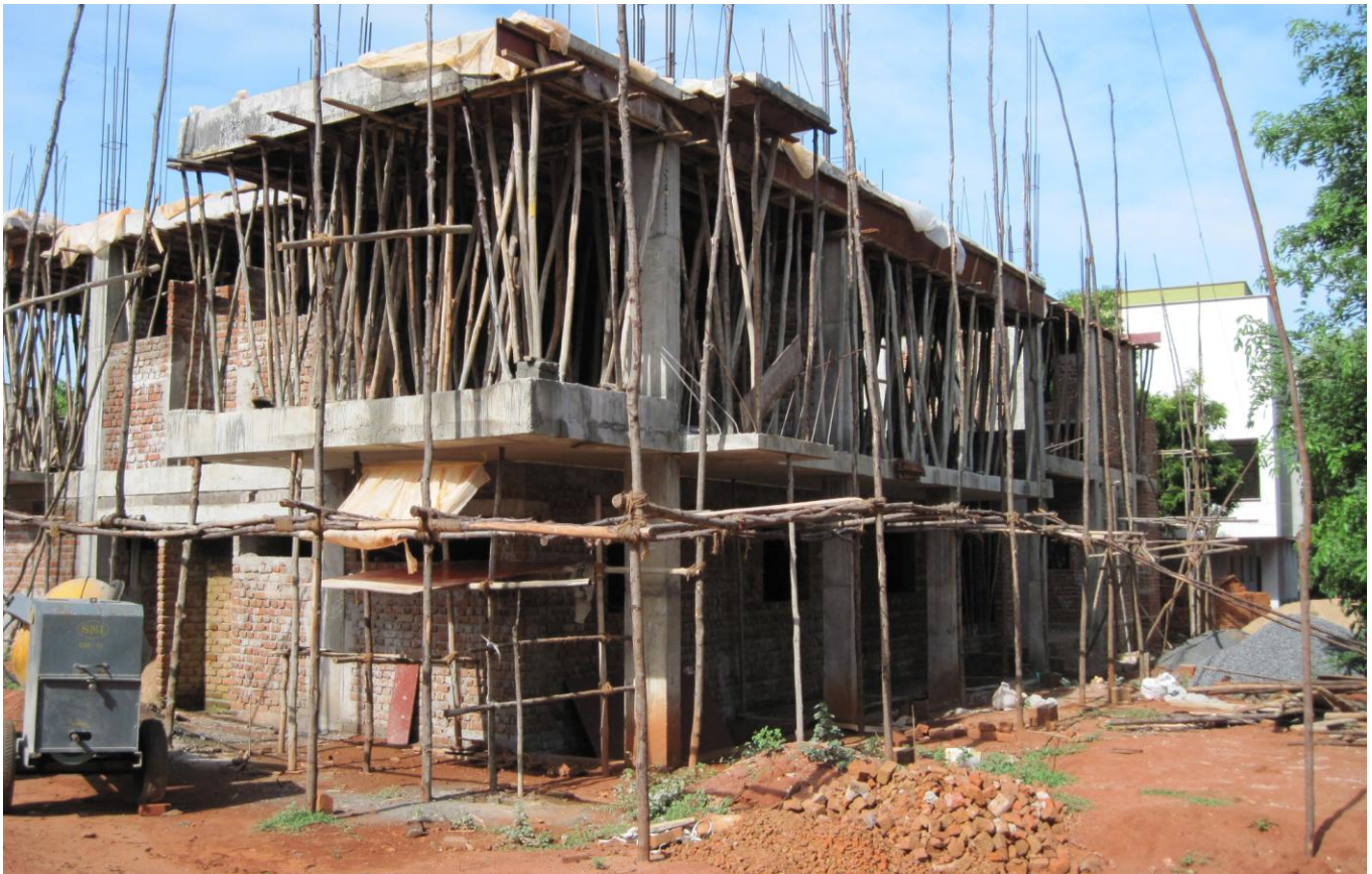
Arati III, Building 2 under construction, estimated finishing time: May 2011
