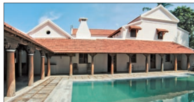
Front views of the Gatehouse before and after restoration. View of the swimming pool in its former backyard.
