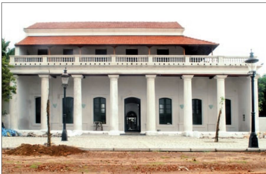
Top: Front view of the restored Bungalow on the Beach; renovated houses in Goldsmith Street; the restored Governor's Bungalow.
