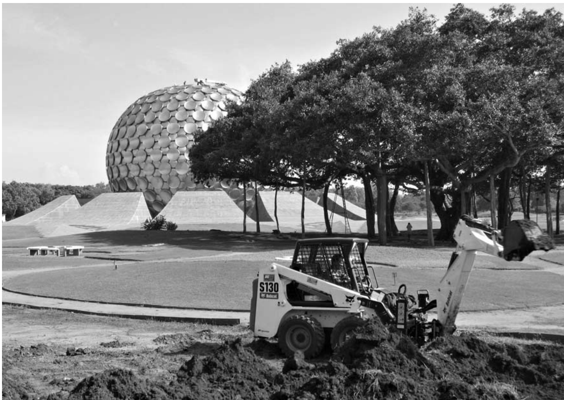
Bobcat preparing soil in the Garden of Unity
