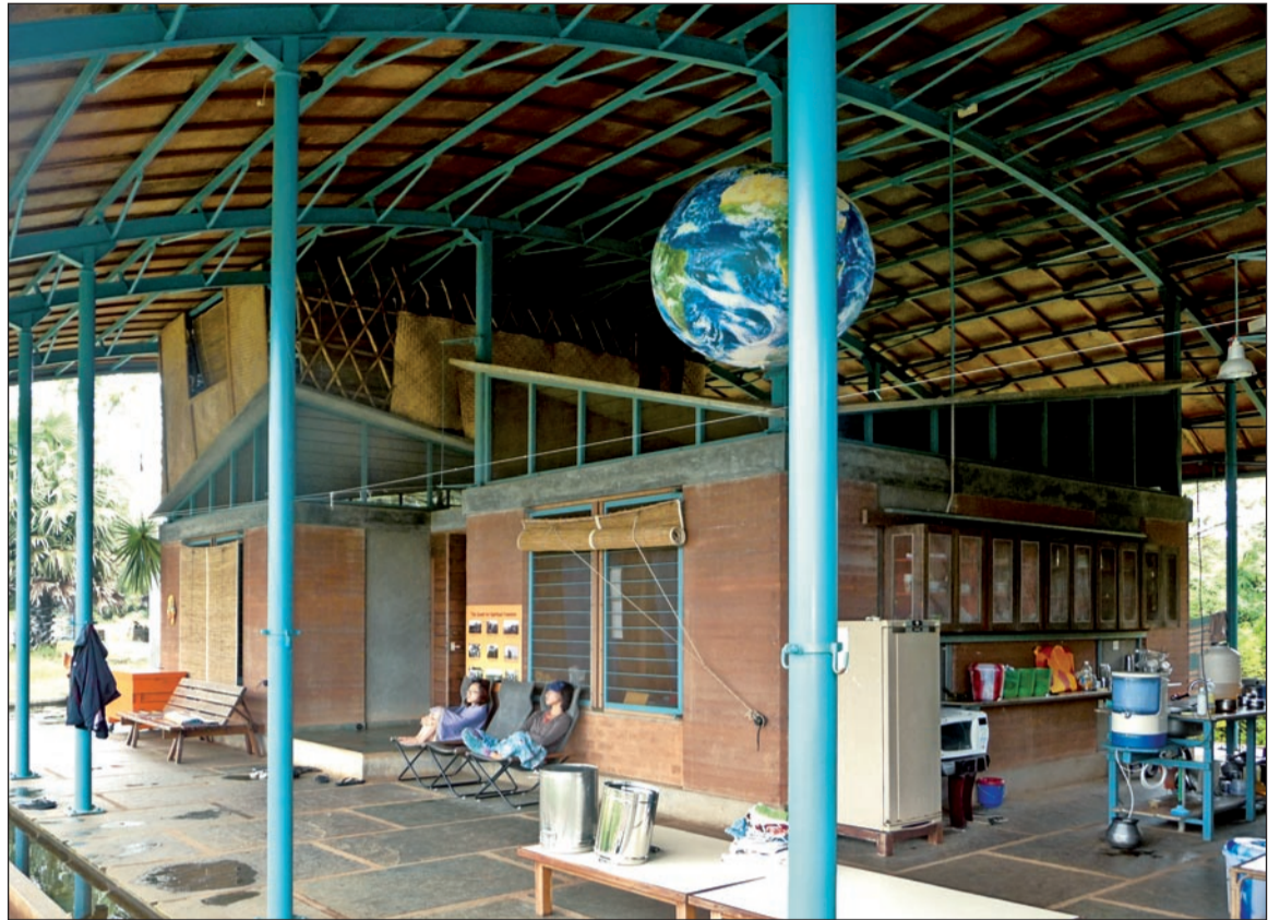
The 'super roof', a steel structure covered in wood, protects the inner dorm rooms, bathrooms and office
