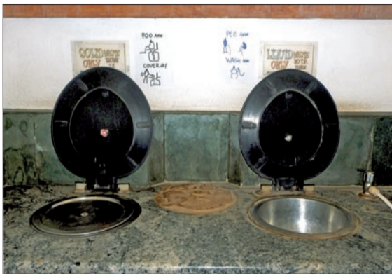
The composting toilets
