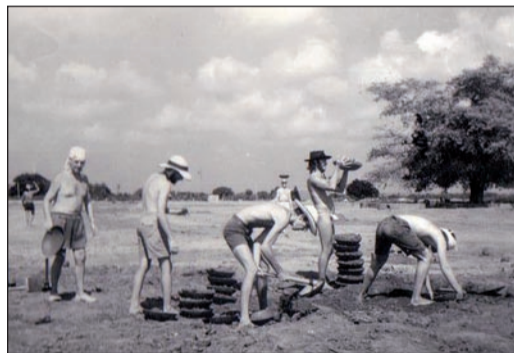
Early Aurovilians starting the excavation.
